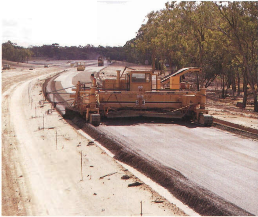
An "autograde" at work on the construction of the Hume Highway at the Seymour Bypass.
